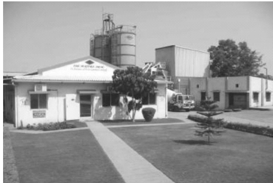
Fig.2 A modern eco friendly RMC plant with advanced manufacturing process and technology for producing quality ready-mixed concretes
