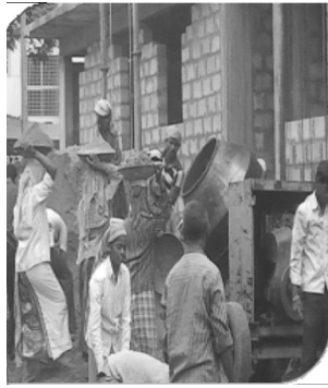
Fig.1 Traditional site mixed concrete under usage in India- the most primitive methods of concreting
