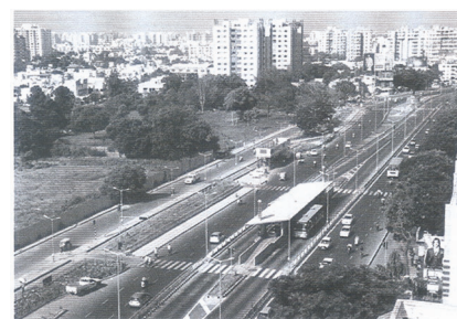
Median bus lane in Ahmedabad (Janmarg)
