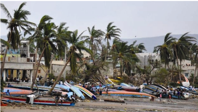
Figure 6. Photograph showing the damage after the cyclone.
