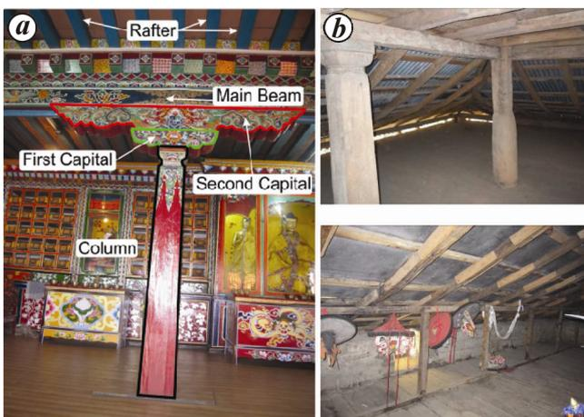
**Figure 4.** Typical details: *a*, Wooden timber frame and floor diaphragm supported on rafters; *b*, hipped roof construction.
