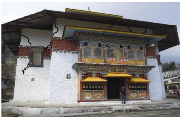
**Figure 8.** Cracks on the exterior wall of Labrang monastery.
