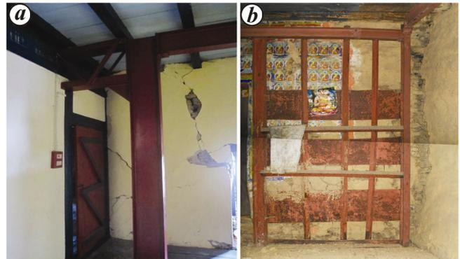
**Figure 5.** *a*, Steel frame in Labrang monastery for retrofitting, which proved ineffective during the September 2011 earthquake event. *b*, Walls damaged by supporting steel structure, Old Ngadak Gompa, Namchi, South Sikkim<sup>4</sup>.
