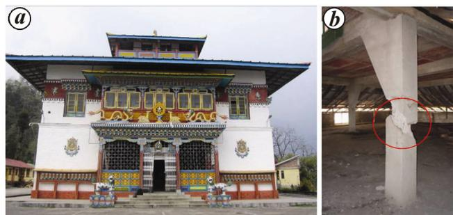
**Figure 9.** a, Phodong monastery, interior RC frame with exterior stone masonry wall. b, Damaged column due to short-column effect induced by the presence of deep haunches.
