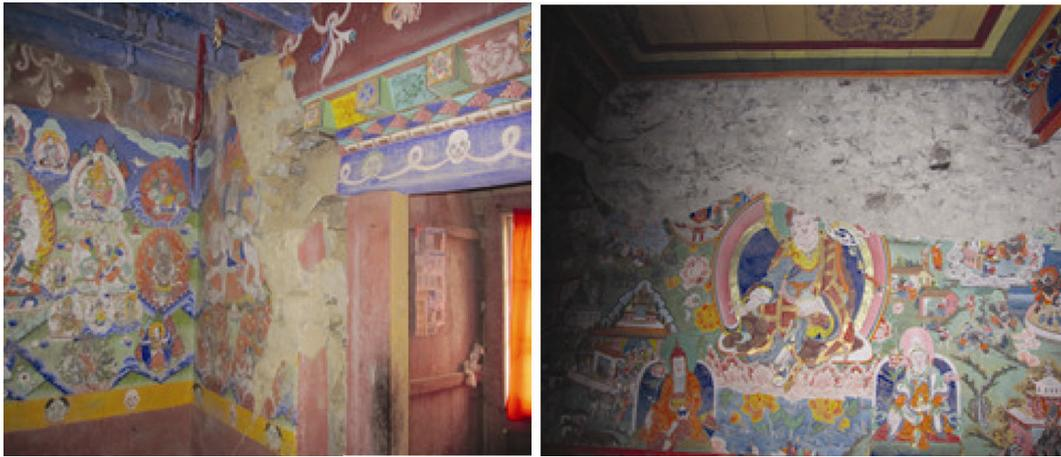
Figure 2. Damage caused to the frescos during the 18 September 2011 earthquake.
