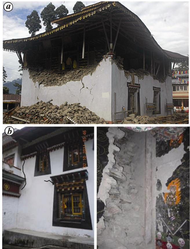
**Figure 6.** Common types of damages observed during the earthquake: *a*, Partial collapse of wall of Ringhem Choling monastery; *b*, Shear cracks and delaminated wall painting at Samten Choling monastery.
