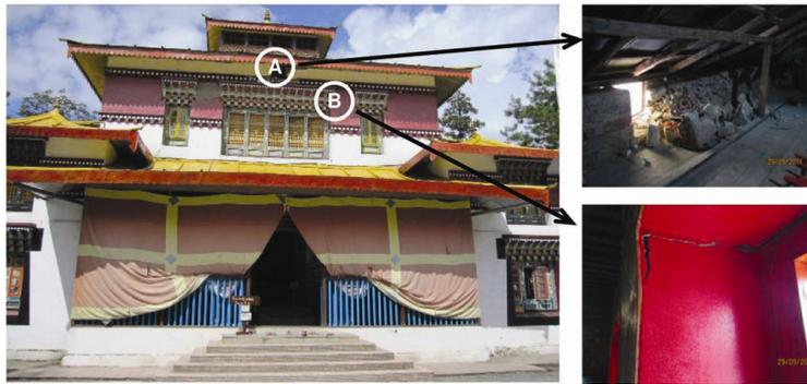
**Figure 7.** Damage observed on the front wall of the third storey at Enchey monastery.
