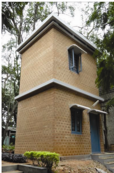
Figure 14. Demonstration building using IOT as fine aggregate.
