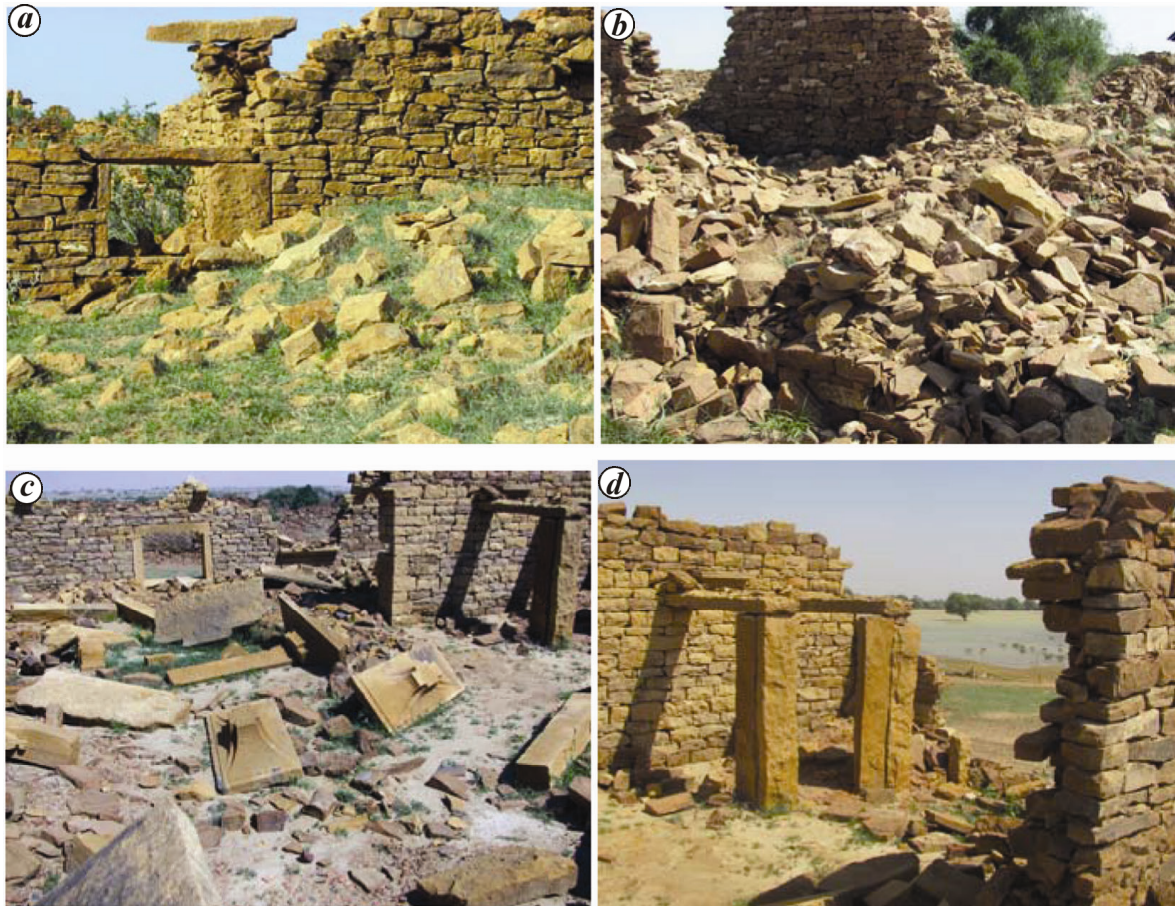
Figure 3 a-d. Collapsed walls and scattered dressed stones along with evidences of fallen joists, lintels and pillars strewn inside the houses. Some collapsed houses turned into heaps of rubble.
