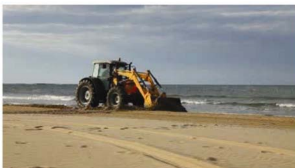
Figure 6. Opening the lagoon mouth mechanically.
