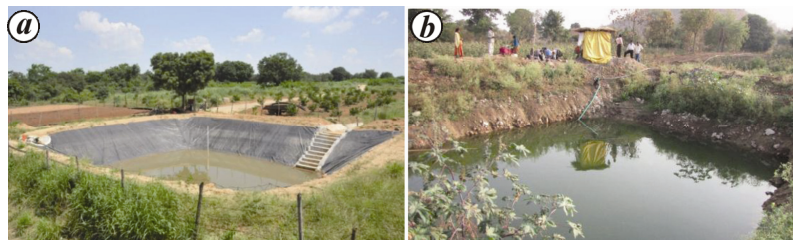
Figure 1. (a) Lined farm pond at CRIDA Farm (red soils) and (b) unlined farm pond in Adilabad district (black soil), Telangana.
