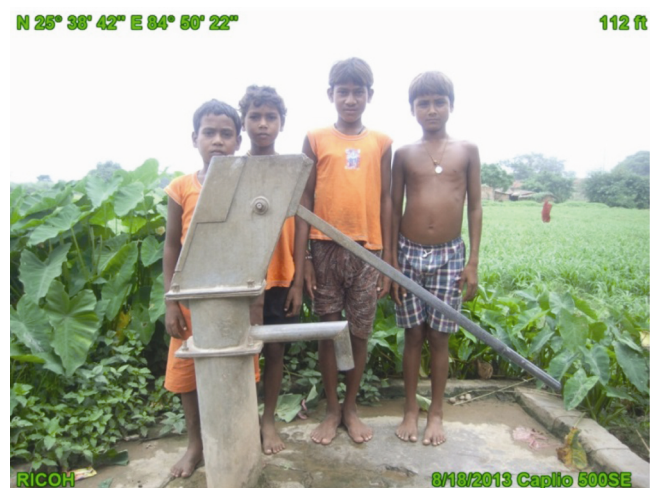
Figure 5. A typical deep tube well installed by the state government (photograph by Sushant Singh, 2013).
