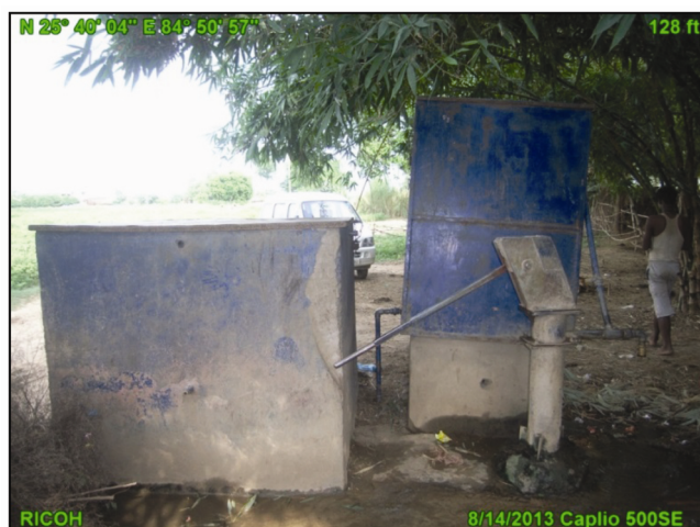
Figure 4. Nonfunctional arsenic-removal unit in Bhawani Tola (photograph by Sushant Singh, 2013).
