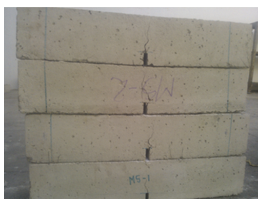
Figure 5. Typical crack pattern.
