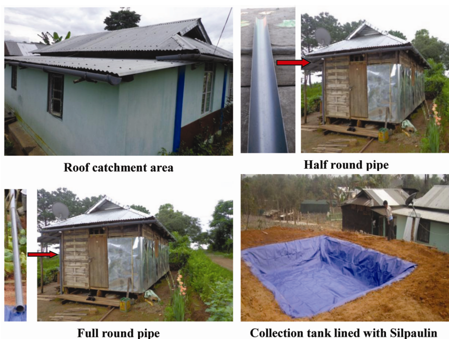
Figure 4. Guttering in roof and lining jalkund with silpaulin.
