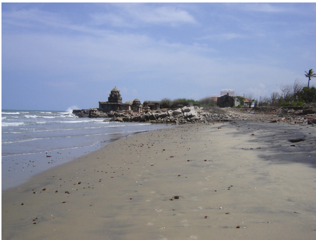
Figure 6. Partly collapsed Masalamani temple in the intertidal zone at Tranquebar.
