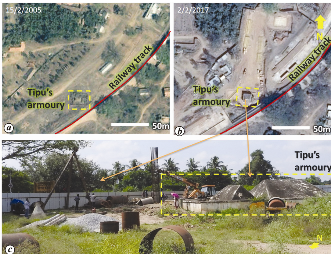
Figure 8. a, b , Google Earth images of Tipu's armoury and railway track. c , Ground photograph of armoury.
