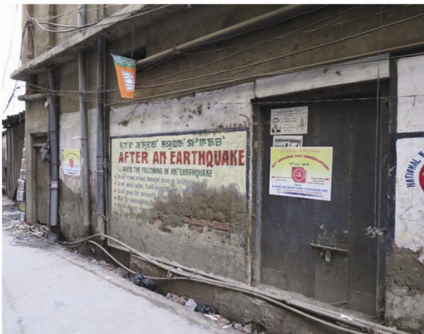
Figure 14. A message on a wall facing street in Imphal reminds that there is earthquake awareness in the region due to frequent shaking.
