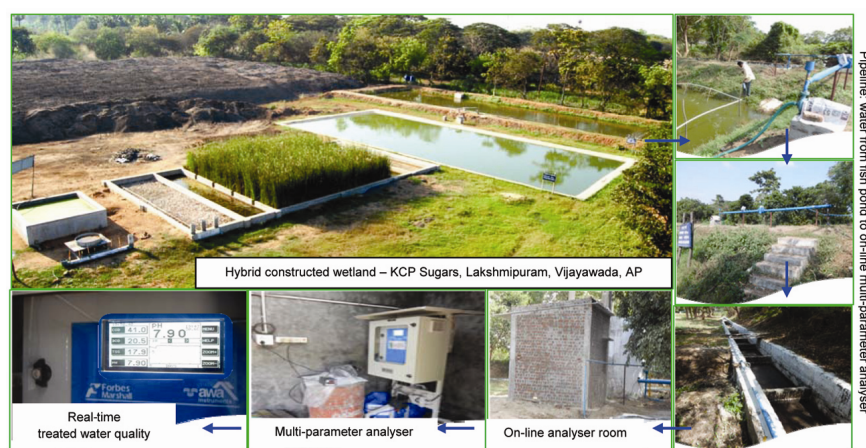
Figure 1. Hybrid flow constructed wetland connected with 24 × 7 on-line monitoring multi-parameter analyser.
