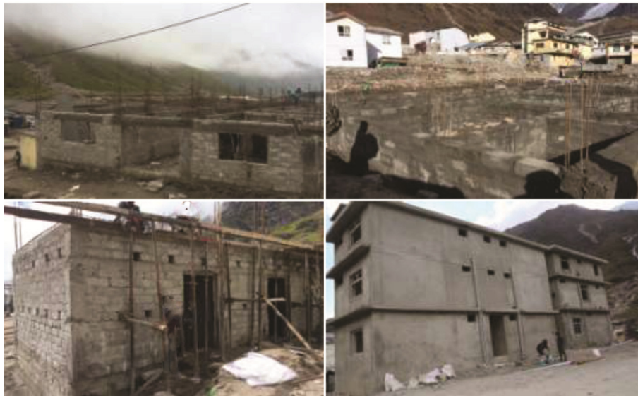
Figure 2. CM construction in Kedarnath post 2013 disaster.
