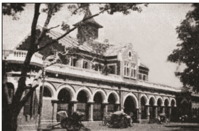
Figure 3. Frontage of the Madras Maternity Hospital (1940s?). Source: https://sriramv.wordpress.com/2015/02/11/government-hospital-for-women-and-children-egmore/
