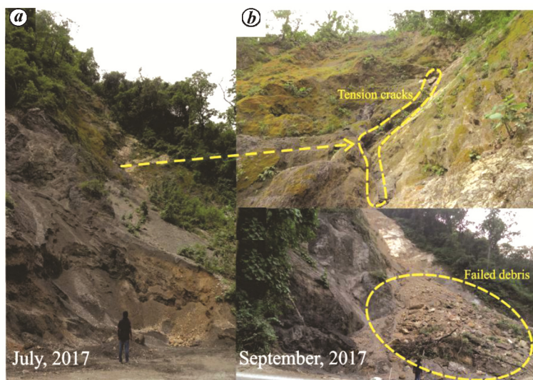
Figure 3. Talus-type slide along NH-58, Shivpuri. a , Pre-failure scenario in July 2017. b , (Inset) Image showing tension crack near crown portion. c , Post-failure condition in September 2017.
