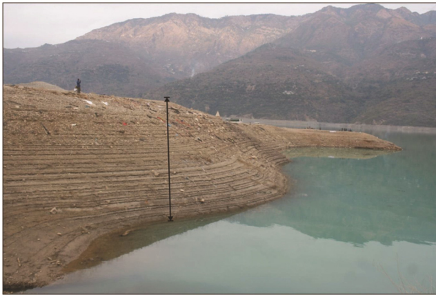
Figure 5. Sedimentological expression of the reservoir level fluctuations that in turn affected the slope instability around the reservoir rim (shown in Figure 6).
