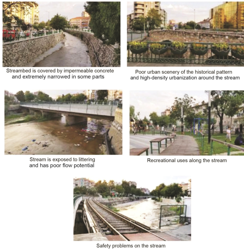
Figure 5. Photographs highlighting the problems related to the Tabakhane stream.
