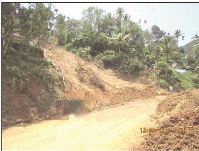
Figure 7. Landslide at Ponmudy S Valavu in Konnathady village.
