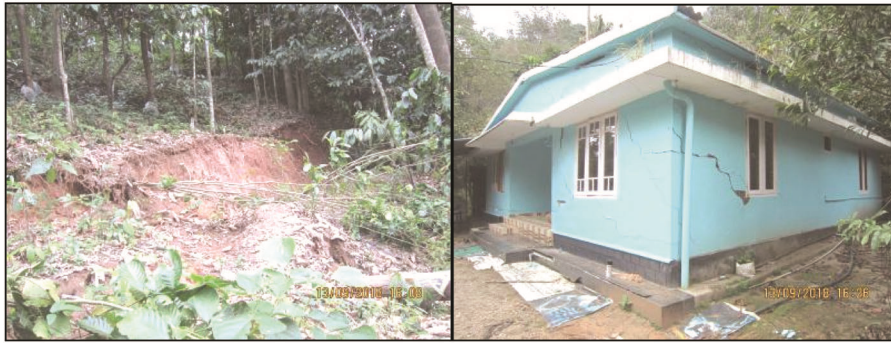
Figure 9. Creep movement in the agricultural land near Viswadeepthi School, Adimaly, Mannamkandom village.
