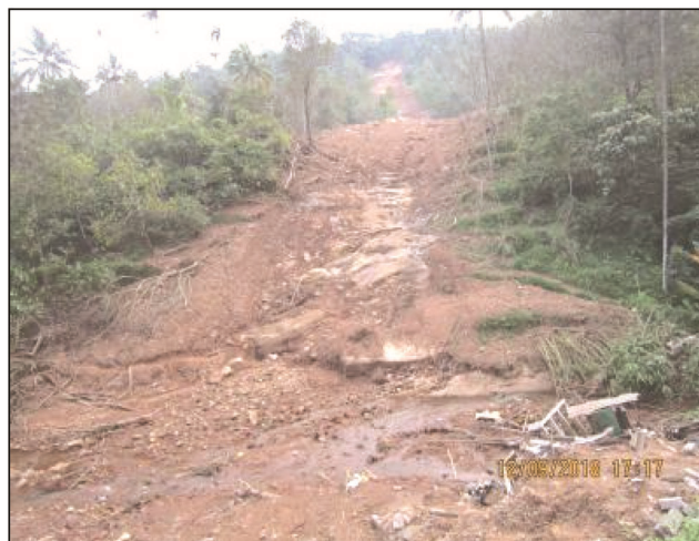
Figure 4. Landslide at Perumkala in Idukki Village.
