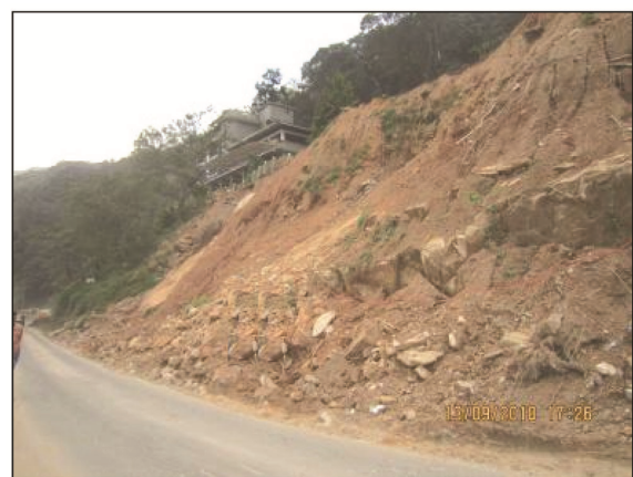
Figure 12. Landslide at 2nd mile in Pallivasal Village.
