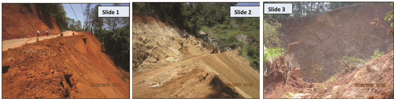
Figure 3. Landslides at Puliyanmala–Thodupuzha Road–Idukki and Arakkulam villages.
