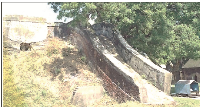
Figure 3. Inclined masonry shaft at Kilpauk, 1872 (photo: N. Meenakshisundaram).
