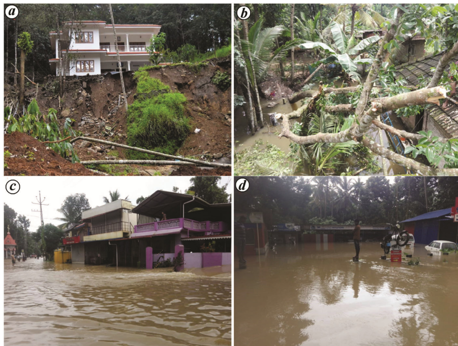
Figure 2. Photographs captured on 9 September 2018 show the devastation caused by the floods in (a) Padanad, (b) Chengannur, (c) Kadapra and (d) Thiruvalla towns in Alappuzha district, Kerala (photos credit: Harsha Rajan).
