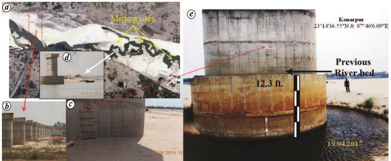
**Figure 6.** River bed incision due to sand mining in Reach 11. *a*, Google Earth Image indicating the location of concrete pillars and sand mining sites. *b*, Photograph of the same pillars. *c*, scale (in ft.) drawn in the base of the pillar ('0' indicate the river bed in 2014). *d*, Sand extracted from the river bed just below the pillars and *e*, Photograph of same pillar in 2017 representing river bed incised about 12.3 ft. in this site.
