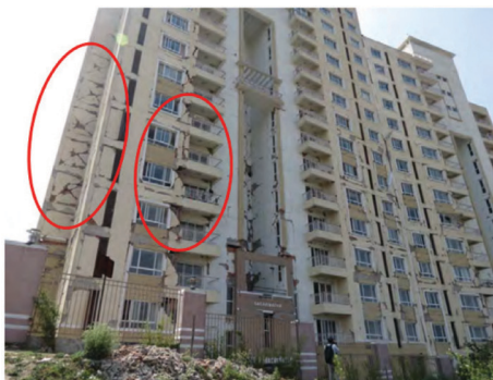
Figure 5. In-plane and out-of-plane damage in a high-rise building during the 2015 Gorkha earthquake, Nepal (image courtesy: Lizundia et al. 10 ).
