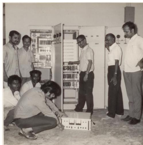
**Figure 3.** Servo system for SLV Radar under test at BARC, Mumbai.
