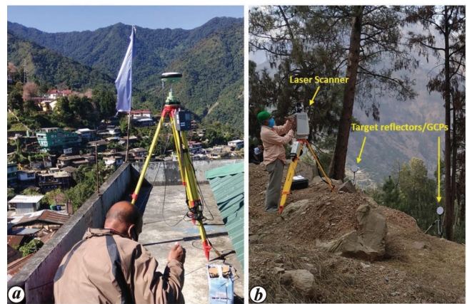
Figure 3. Components of data acquisition. a, GNSS base station set up on a rooftop at Phesama, Nagaland. b, Field scanning conditions illustrating setting up of target reflectors.
