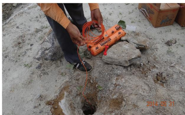
**Figure 3.** View of explosive charging of holes with Handydet 400/25 ms delays.
