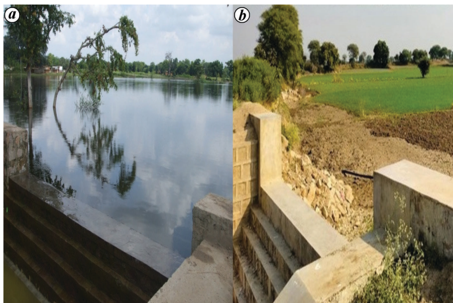
Figure 2. a , Harvested water in the Haveli during monsoon season. b , Cultivated Haveli bed during post-monsoon season.
