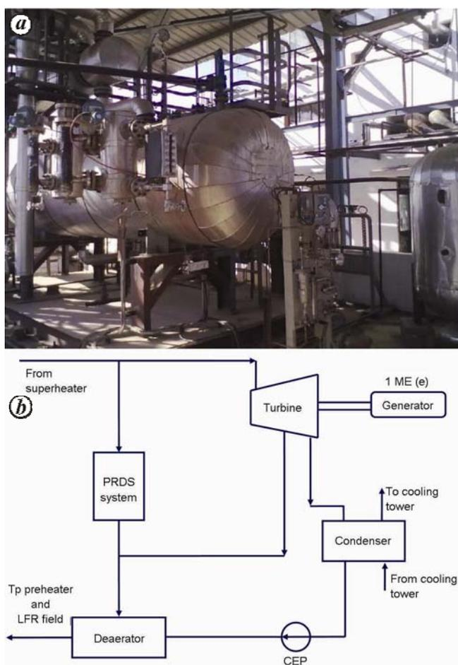
**Figure 5.** a, Heat exchanger installed at site. b, Schematic diagram of power block.
