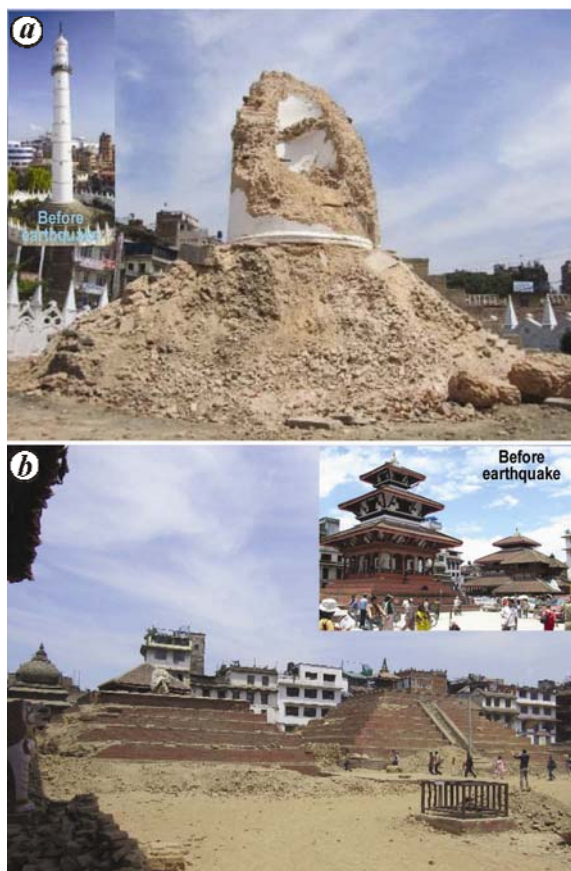
Figure 4. (a) Collapse of Dharhara tower in Sundhara, Kathmandu ( 27^{\circ}42'3'' , 85^{\circ}18'42'' ). (Inset) Before earthquake (photo: Corbis Ian Trower). (b) Collapse of temples in Hanuman Dhoka, Kathmandu ( 27^{\circ}42'14'' , 85^{\circ}18'29'' ). (Inset) Before earthquake (photo: Andrej Pauš).
