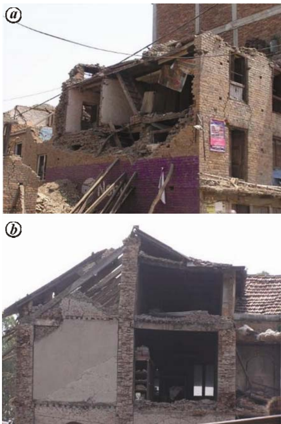
Figure 7. Typical out-of-plane failure of unreinforced masonry walls: (a) Failure due to absence of positive connection between the cross wall and main wall in Nikosera (27°40'45", 85°24'10"), and (b) failure due to proper connection between floor/roof diaphragms and walls.
