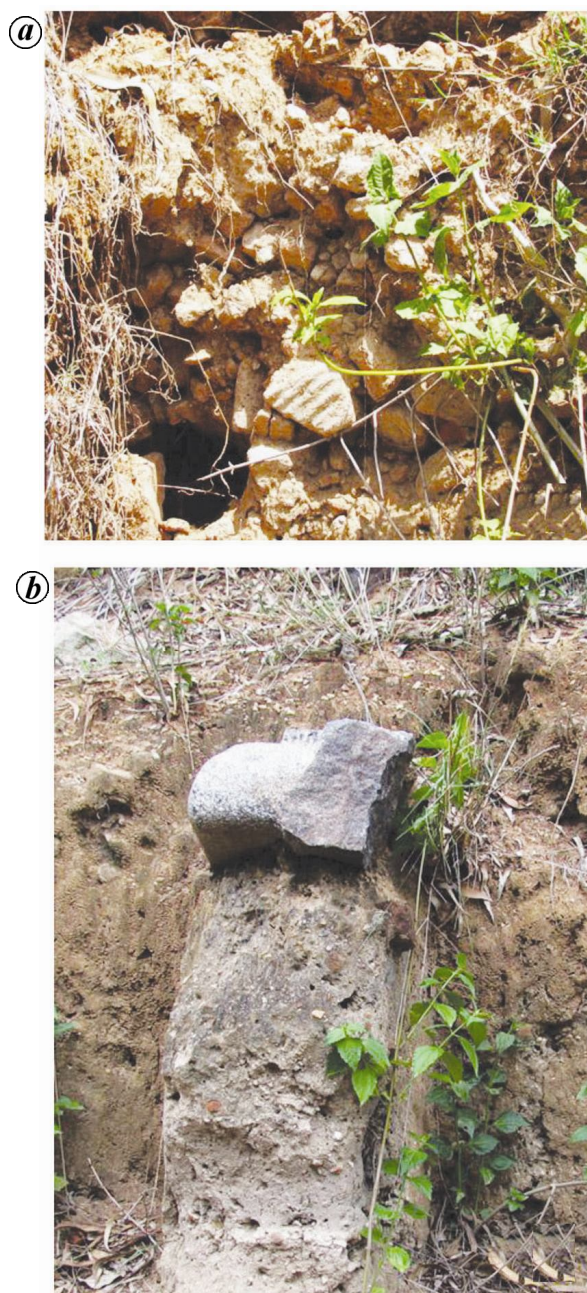
Figure 13. a , Earthquake debris mixed with soil. b , A broken piece of plinth lying over flood plain deposit mixed with earthquake debris.
