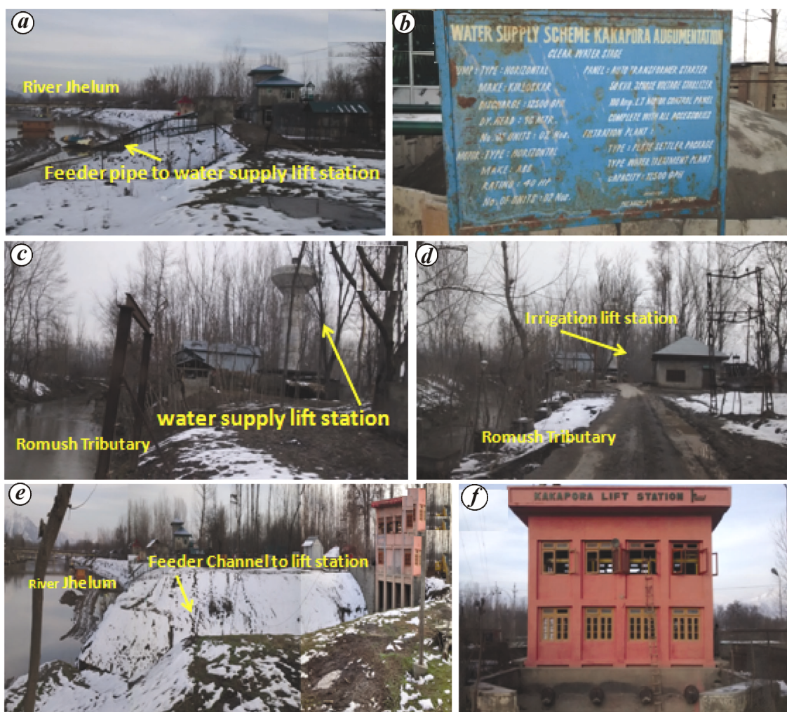
Figure 7. Field photographs during low flow period showing water supply schemes ( a, b ) at site S13 (Kakapora) on main River Jhelum and ( c ) S14 (village Gundipora) on Romush nala. Irrigation lift stations at ( d ) S14 (village Gundipora) on Romush nala and ( e, f ) site S13 (Kakapora) on main River Jhelum. Romush nala is a major tributary of River Jhelum. Schemes are established to supply water for domestic (including livestock) and irrigation purposes in the valley.
