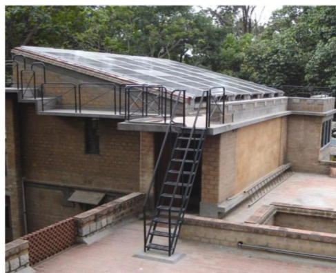
Figure 5. Design of climate-responsive building (left) with integrated PV roof (3 kW) at the Centre of Sustainable Technologies, Indian Institute of Science in Bangalore 2 .
