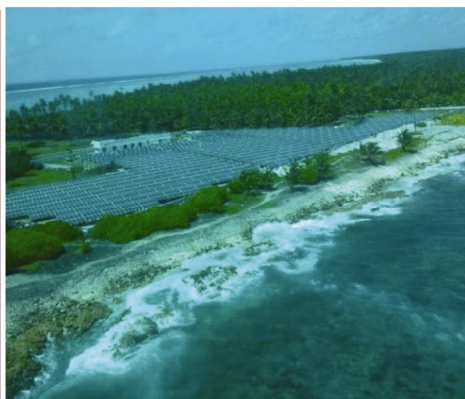
Figure 7. (Left) Schematic diagram of hybrid power system (wind–diesel–solar PV). (Right) Kavaratti island: Single largest solar plant among 11 Lakshadweep islands; 760 kWp solar PV-cum-diesel hybrid power plant; Eco-friendly; Diesel saving/day ~1000 liters; Commissioned: October 2011.
