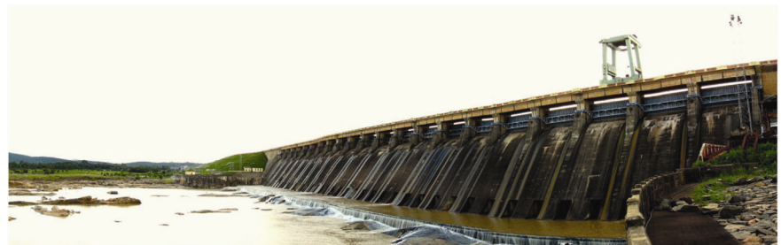
Figure 2. Hirakud dam, Odisha 4 .
