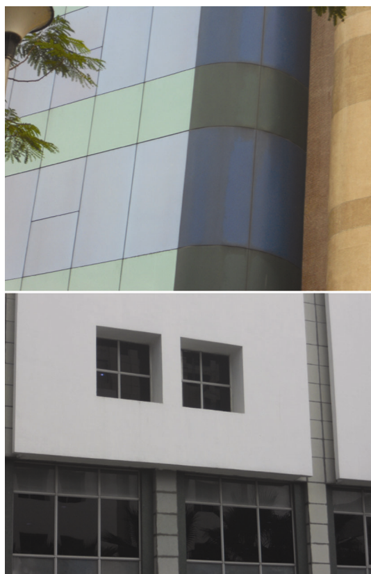
Figure 4. Facade of office building of Firm A (glass curtain wall) and Firm B (window).
