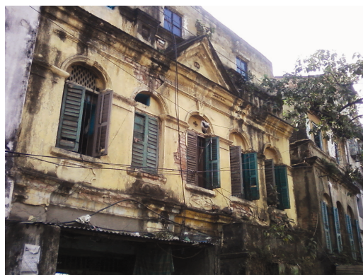
Figure 2. Louvered timber windows of an old building.
