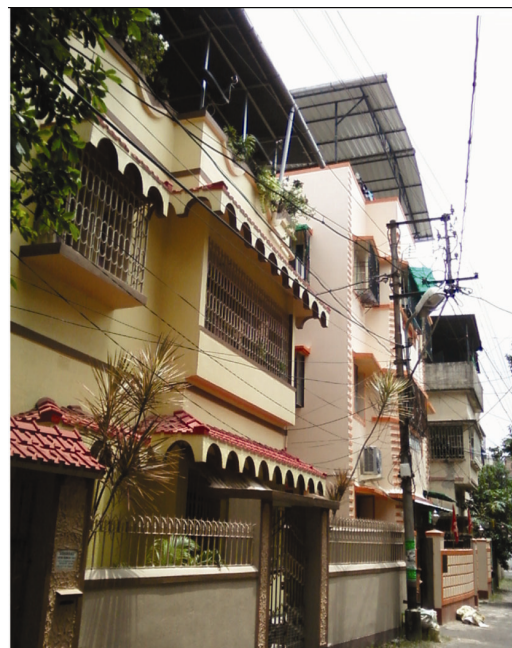
Figure 5. Low-rise buildings with GI-sheds over the roof.
