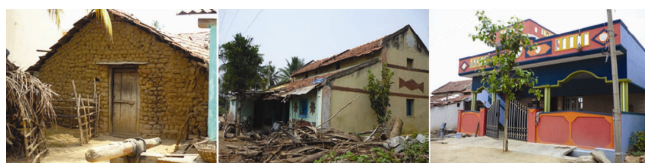
Figure 2. A sample of building types in Ungra village. (Left) Gabled roof adobe house, (Middle) Gabled roof brick-plastered house with verandah, (Right) Flat roof concrete dwelling with compound wall and parking space.
