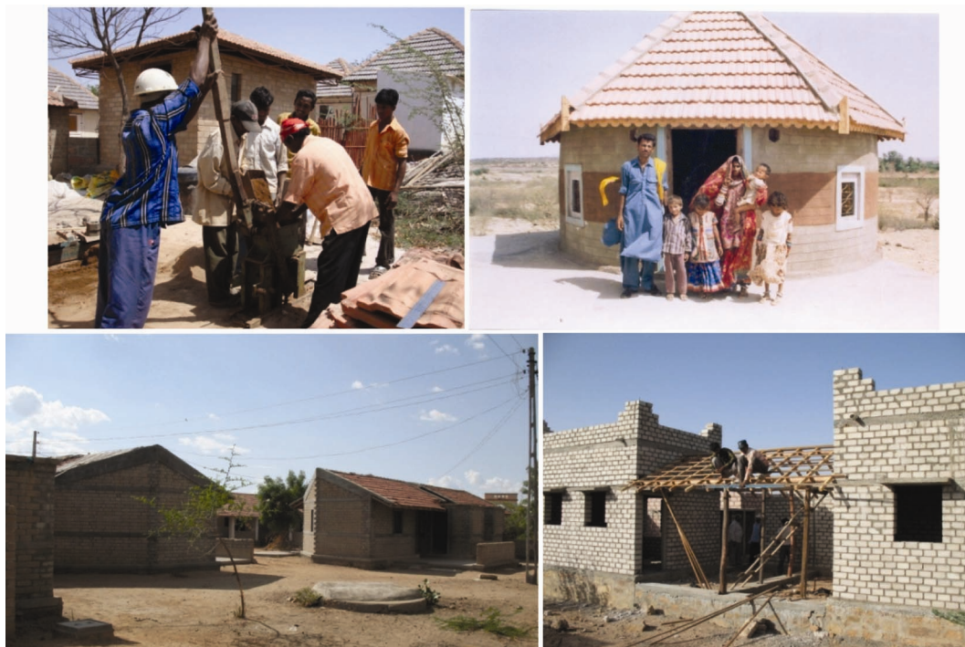
Figure 14. Block making and stabilized soil block houses.
