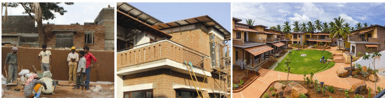
Figure 16. SSB production at site and SSB masonry houses.
