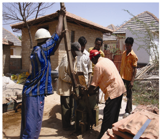
Figure 8. SSB block production using manual machine.
