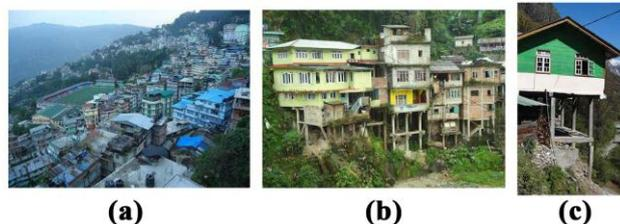
**Figure 1:** RC frame building in hill slopes built in last 10-15 years (a) Skyline of Gangtok city; (b) Building that lack many desirable earthquake resistant feature; (c) Building that lack many desirable earthquake resistant feature
