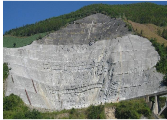
(b) After reinforcement
