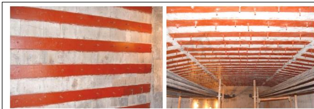
Figure 5: The web and roof strengthening
