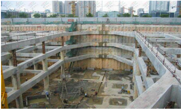
Figure 2: The supporting structure of a deep foundation pit
