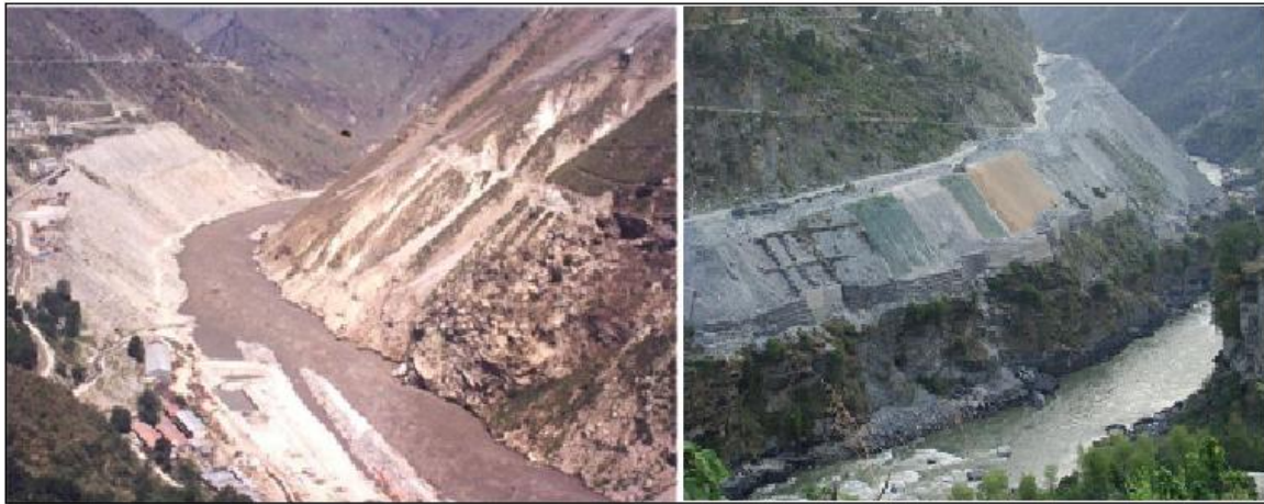
Picture 2. Disposal of Excavation/Construction material along Satluj River in the Study Area
