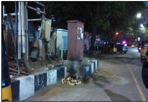
Figure 15: Obstruction in the form of Electric Board (EB) in Reach 1 B
