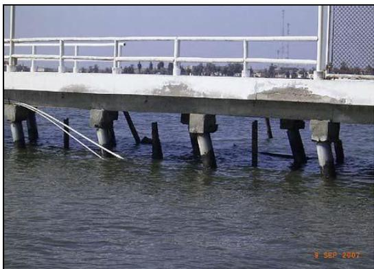
**Figure 2.** Jetty structure damaged at Yacht Club in Paracas during 2007 Peru earthquake
