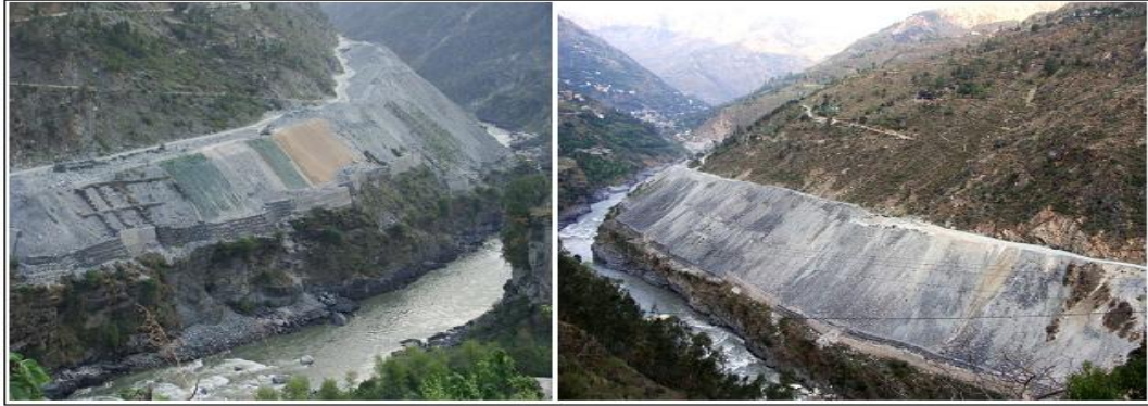
Fig.6. Disposal of Excavation/Construction material along Satluj River in the Study Area
