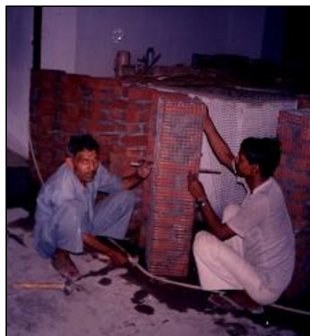
Figure 5. Wire mesh encasement of brick column in progress
