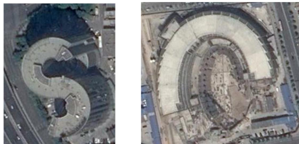
Figure 9. Some peculiar building outlines.
