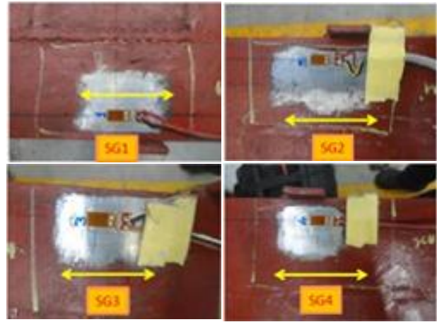
Fig. 11: Linear gauges installed on the platform
