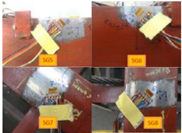
Fig. 12: Rosette gauges installed on the platform
